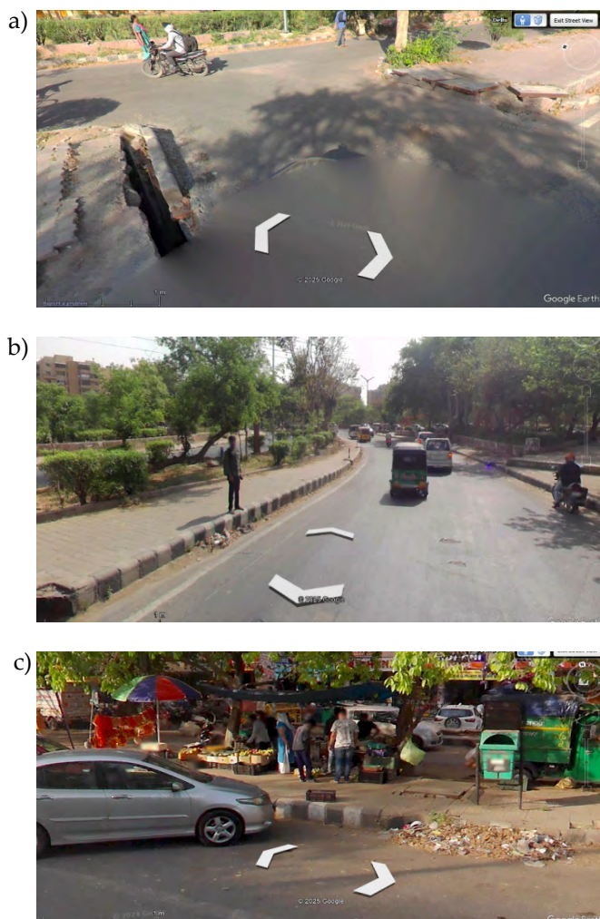
Fig. 4. Lack of maintenance near Ayudhvihar Chowk (a); footpath too high and no marked pedestrian crossing near Sector 3, Aastha Kunj (b); lack of cleanliness, vendor encroachment on footpath near Aashirwad Chowk Market and access to footpath partially blocked (c)
